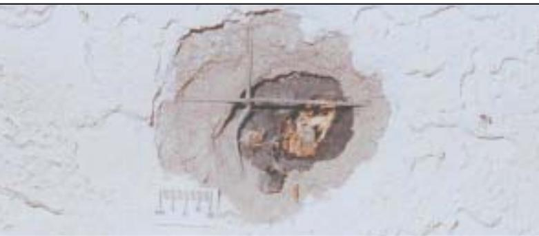
Above photo shows exit point of stucco wall after bullet has passed through corner (i.e. two complete walls).
